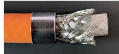
Figure 26: shorten the shielding
